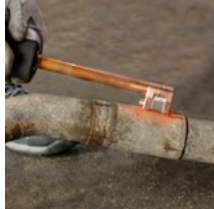
Removing exhaust pipes
